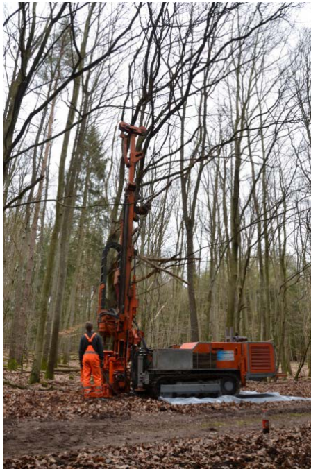
Drilling of groundwater wells at Lake Hinnensee
