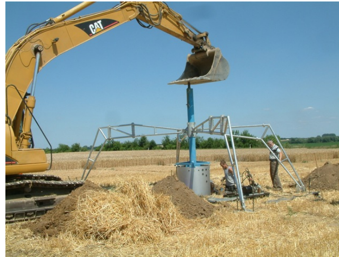
Construction of a lysimeter at Dedelow
