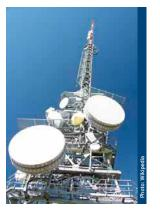
Precipitation data is often collected with the help of socalled 'rain gauges'. The new method being tested by the PROCEMA project makes use of microwave links run by mobile network operators (image right: a radio tower). The in-house developed measurement device can also calculate integrated absolute humidity
